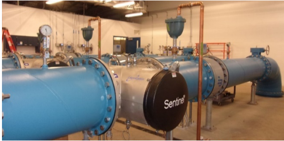
UV reactors treat the water to achieve LT2 compliance
