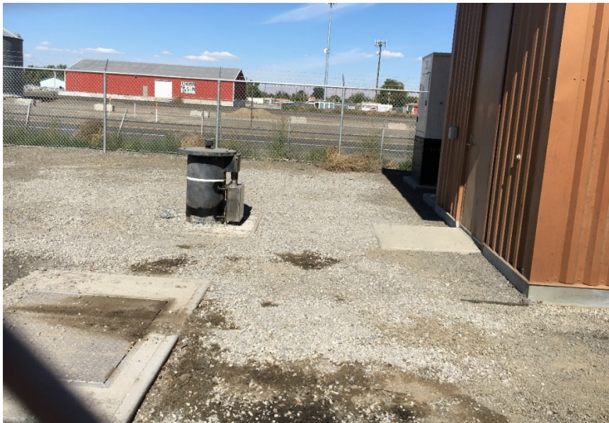
New well, control building, and generator.
