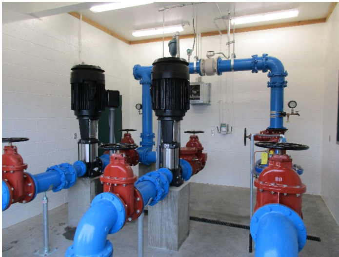
New booster pumps
