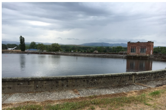
Mill Creek raw water basin
